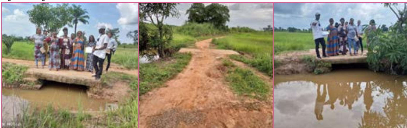
Figure 6 Imogo Amaeze Culvert Visuals.
