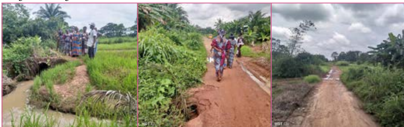
Figure 1 Uhuogiri Culvert Visuals
