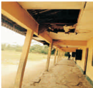
Broken floor & Ceiling at CPS II Sagbama
