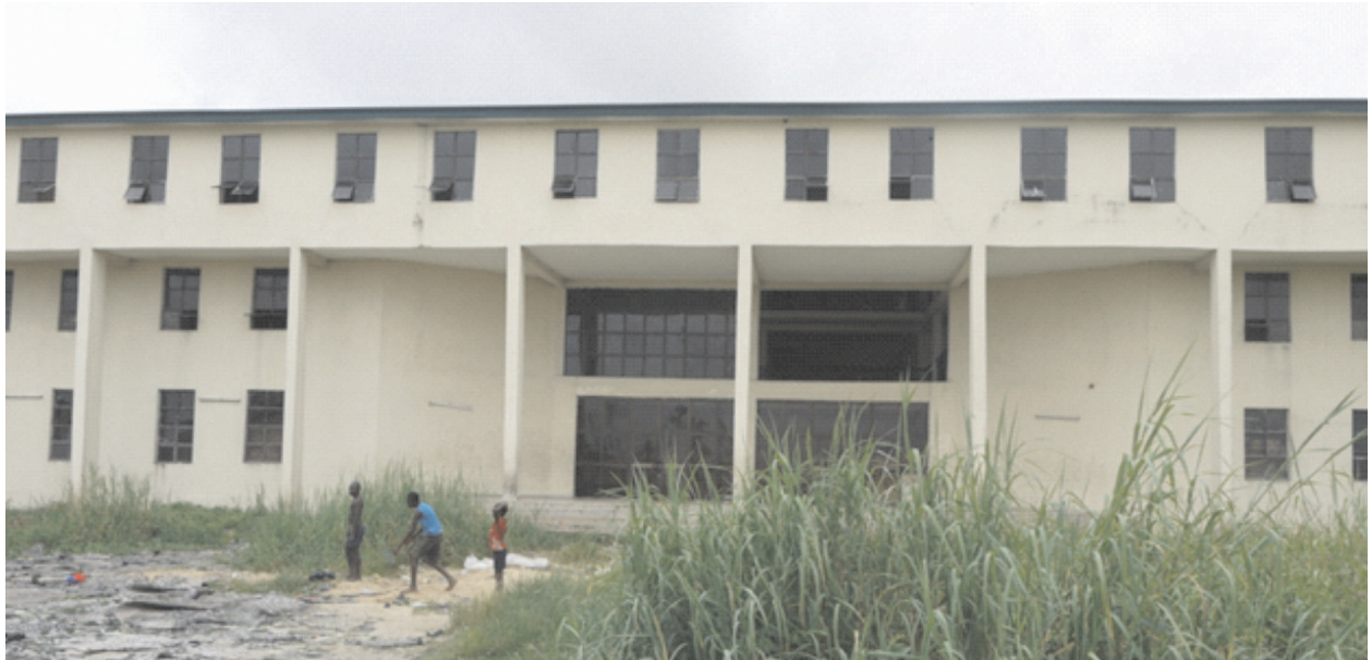
Construction of Senatorial Model Secondary School Yenagoa.
