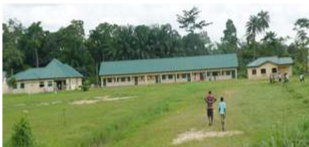
Rehabilitated Nembe National Grammar School
