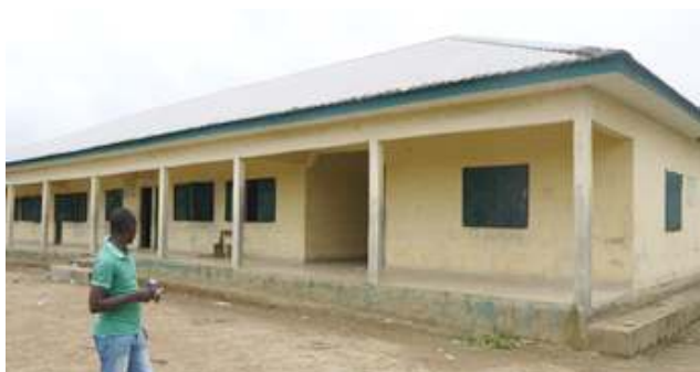
BJSS Igeibiri Southern Ijaw LGA. No Rehabilitation or Repairs
