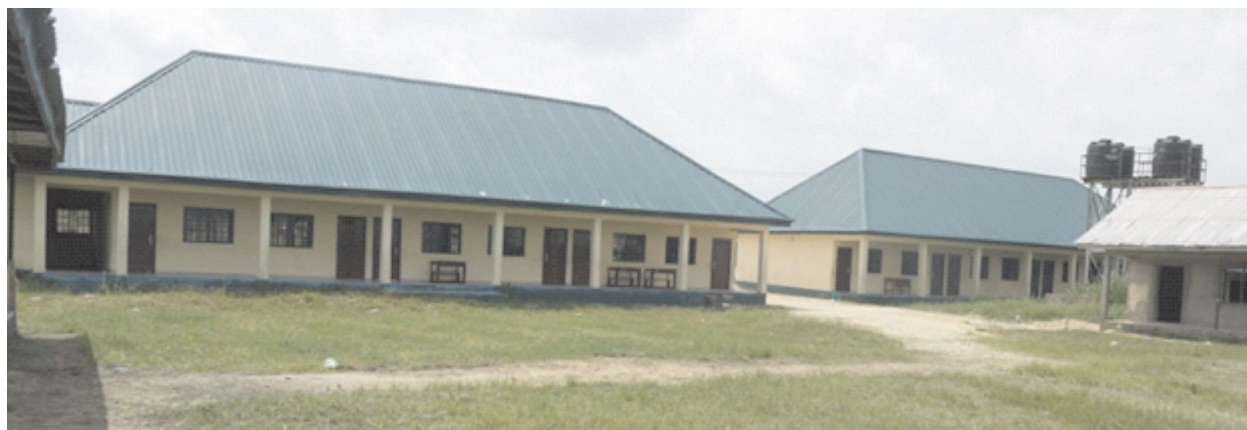
Some renovated Classrooms blocks at CPS Toru Orua
