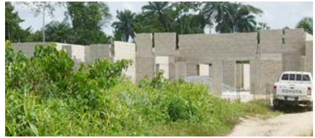
General Referral Hospital Ogbia. Ongoing construction work at very slow pace
