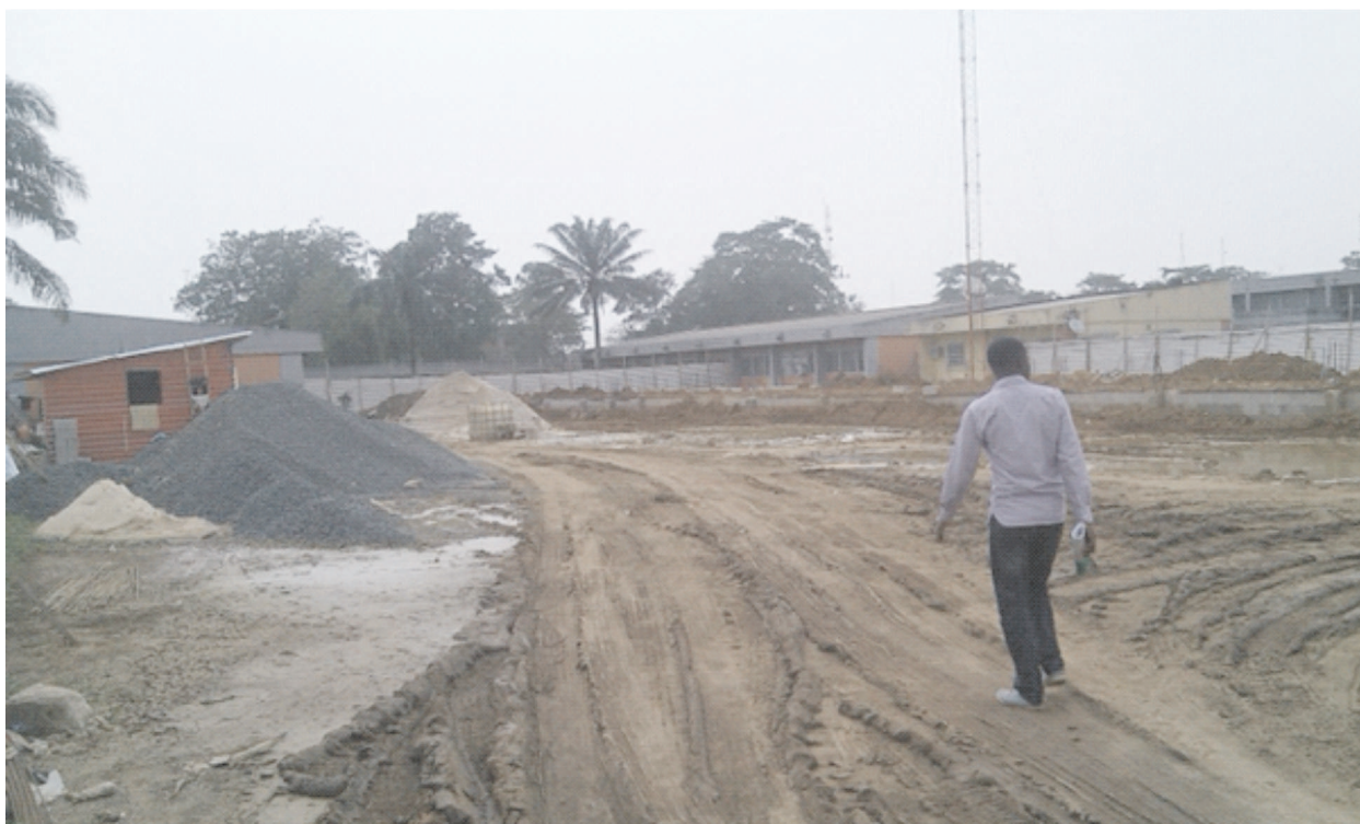
Construction of Laboratory, Marine Engineering Department, RSUST
