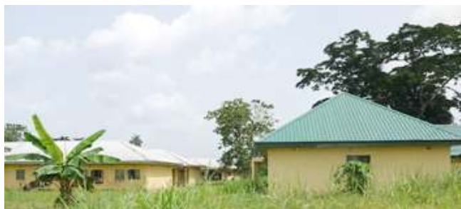
CSS Angalabiri. No Rehabilitation or Repairs
