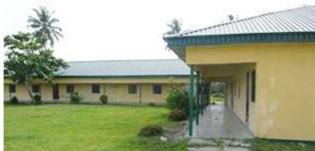
CCSS Opume had already been renovated by ETF IN 2011.
