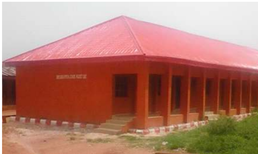
New construction at Iyoba School of the Gifted
