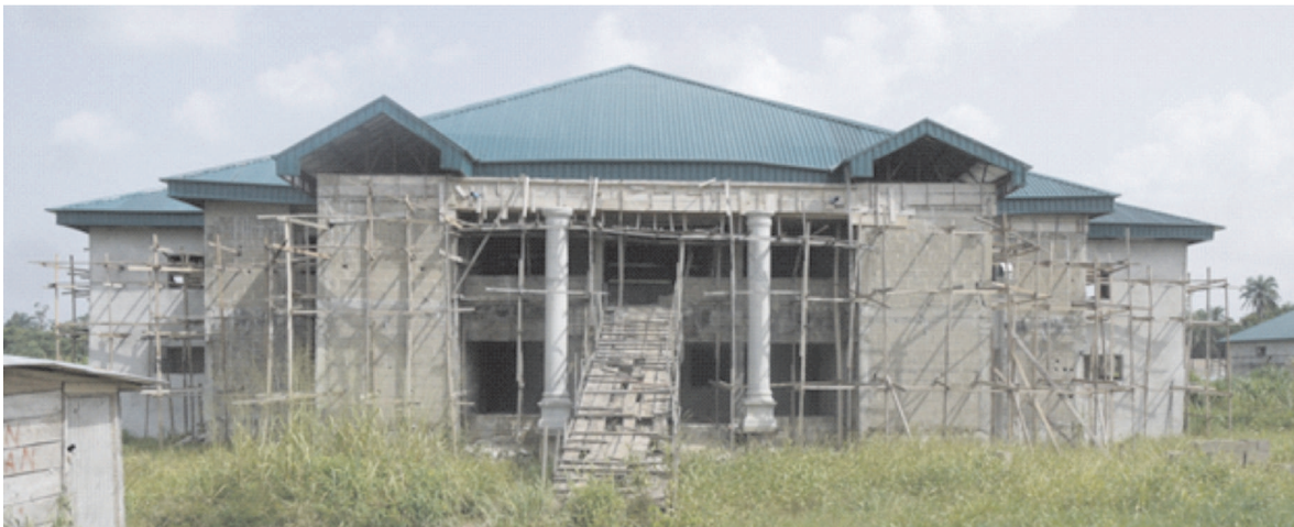
Ongoing Construction at Isaac Jasper Boro College of Education
