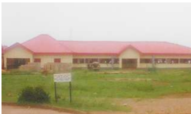
Newly Constructed classroom Block, Ihogbe School
