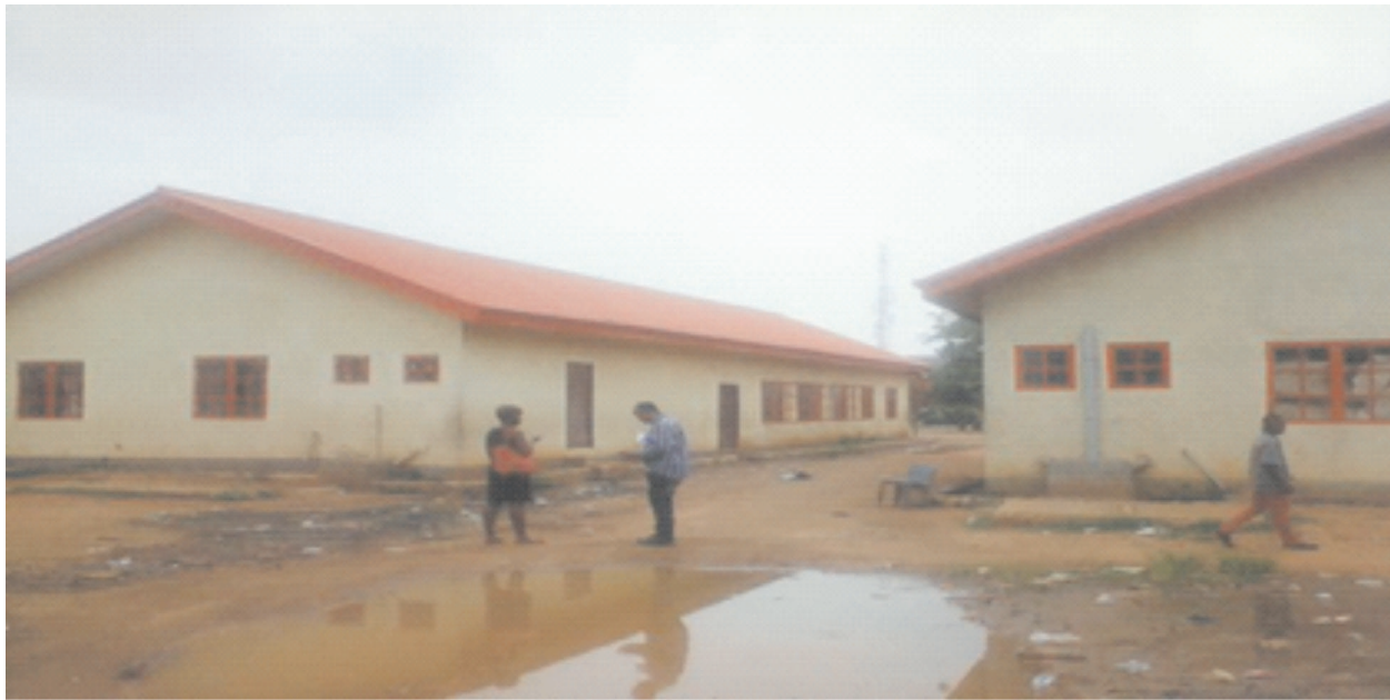
New construction at Oba Akenzua Secondary School
