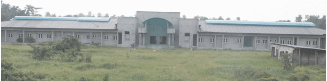
The Referral General Hospital Sagbama. Abandoned and overgrown with weeds
