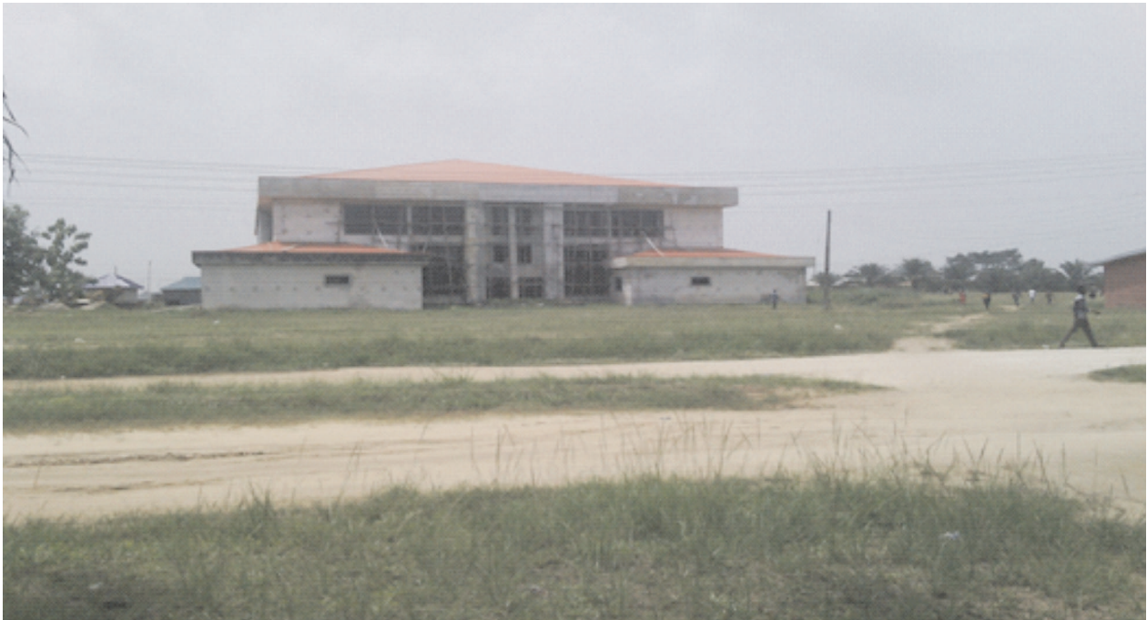
Auditorium under construction at Ozoro Polytechnic, Ozoro
