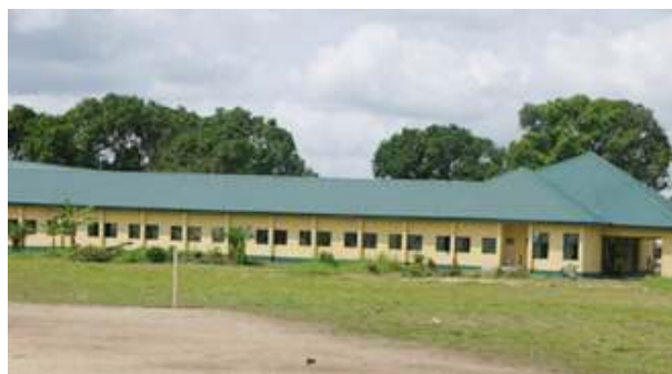
GGSS Ogbia town. Rehabilitation/Repairs works were carried out in 2014
