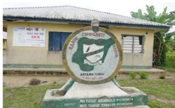
CPS Anyama and Tarakiri Community Secondary School. No Rehabilitation or Repairs
