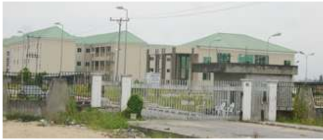
Chief Melford Okilo Memorial Hospital. Construction work resumed after over 4 years of pause.
