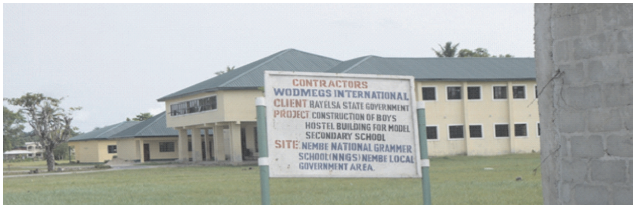
Ongoing Construction of Model Secondary School Nembe
