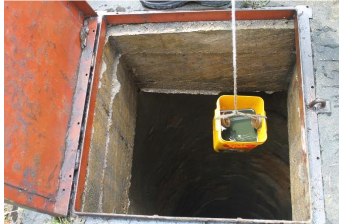
Crude oil storage pit
