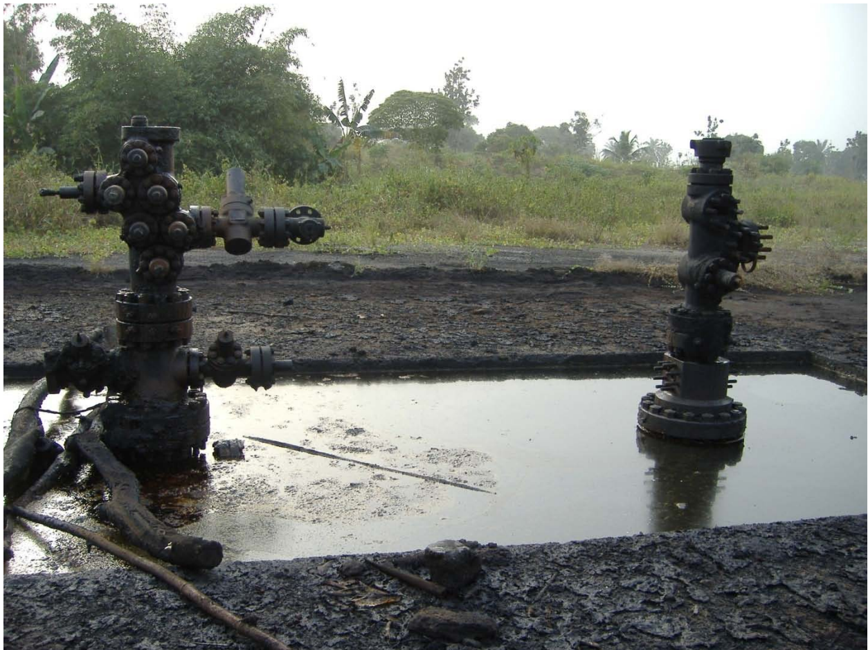
Oil installations like this one have polluted farmlands in Ogoni
