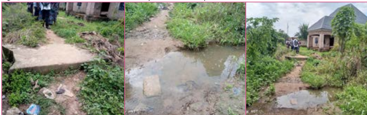
Figure 8 Old Ibe Abbah Culvert constructed far away from the water way and rendered redundant
