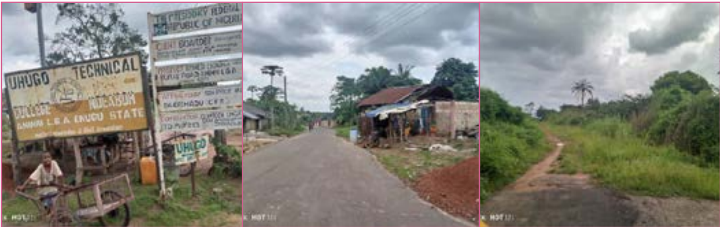
Figure 5 Ezinesi Ndeaboh road; from the beginning to the end
