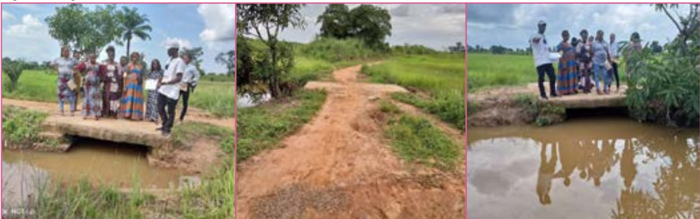
Figure 6 Imogo Amaeze Culvert Visuals.
