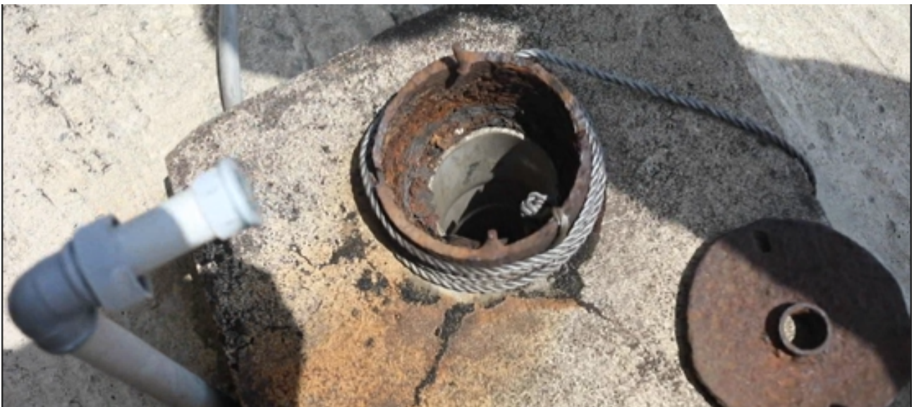
Abandoned primary school borehole, contaminated by gas leakage from the soil
