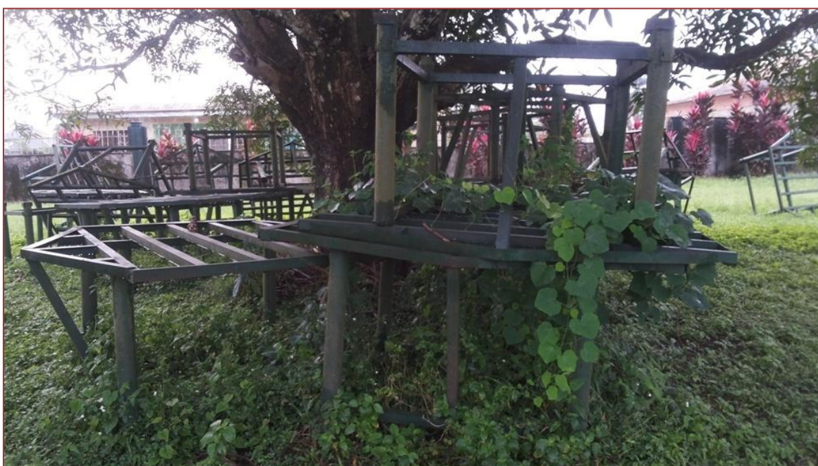
Figure 9: Water tank stands are seen abandoned in Khana LGA
