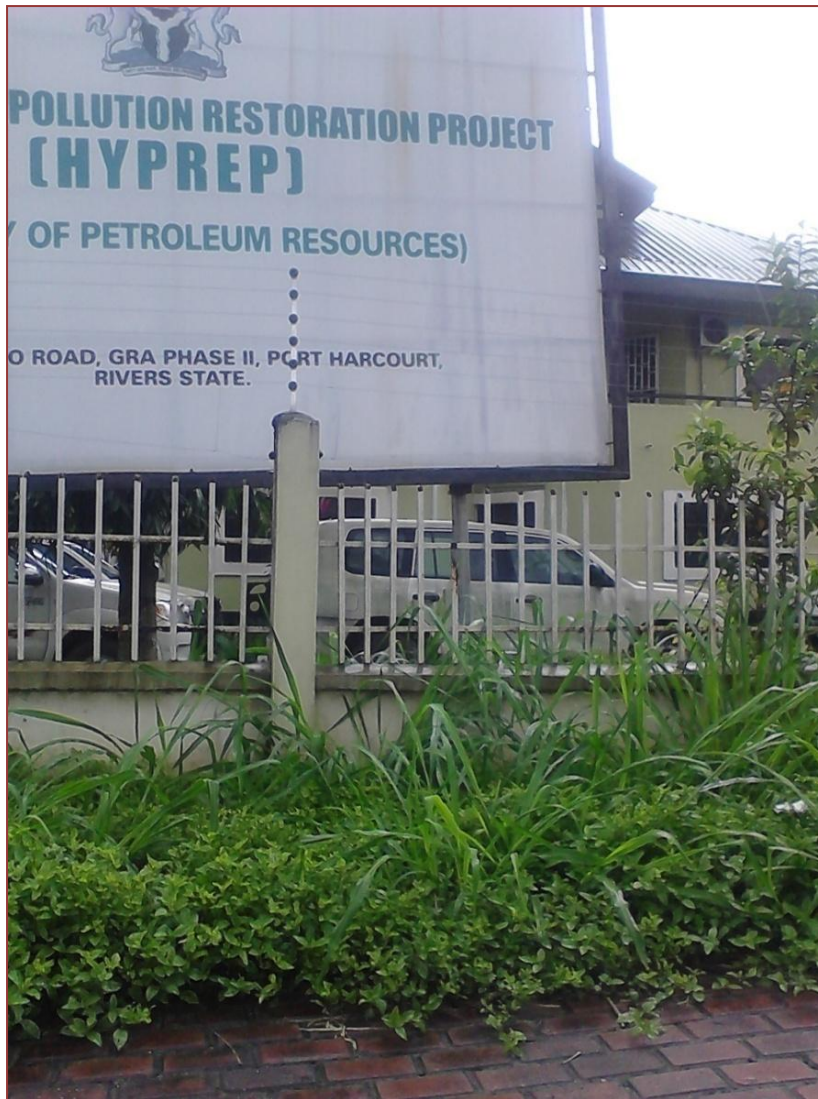
Figure 4: HYPREP office in Port Harcourt is abandoned
