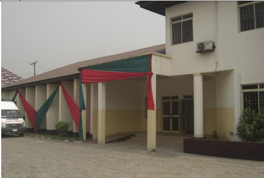
Primary Health Centre, Borokiri, Port Harcourt as at January 2011
