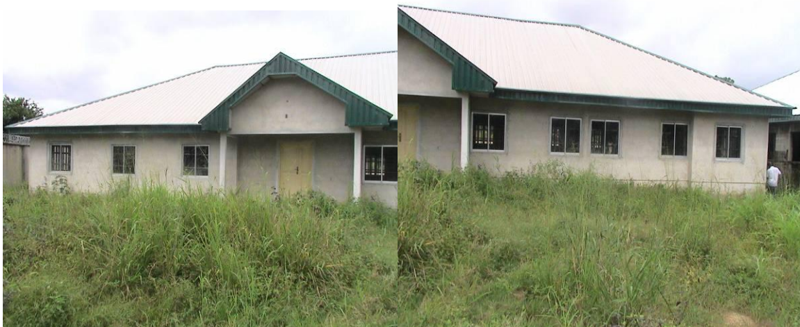
Primary Health Centre, Mbiabong Etoi as at October, 2010
