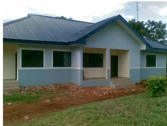
Newly constructed Staff Quarters at the Health Centre
