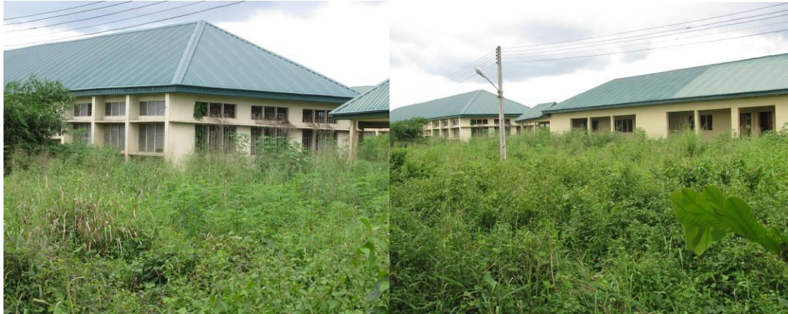
Abandoned Model Secondary School Construction, Ekparakwa as at October 2010
